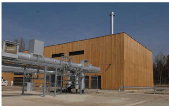
Type of plant: hydrothermal doublet Drilling depth: 4,083 metres (production borehole), 4,453 metres (re-injection borehole) Installed thermal capacity: 50 MW Installed electrical capacity: 4.5 MW
